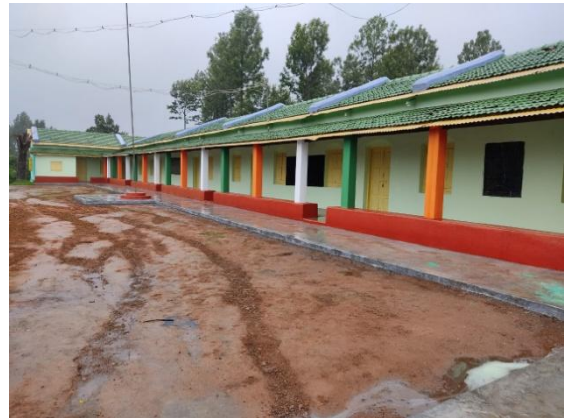
SCHOOL READY FOR REOPENING
