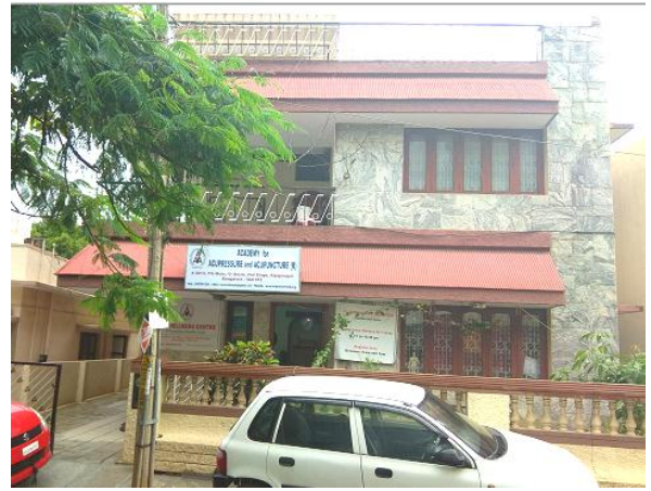
The Commercial building identified by Dr. H. Bhojraj in 2017
